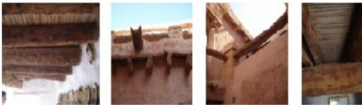
**Fig. 4.** Various uses of palm trees: beams, gutters, fences, and false ceilings<sup>29</sup>.
