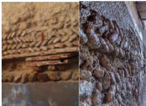
**Fig. 3.** Mixed walls with double layer of terracotta brick and rubble-medina of Tlemcen.
