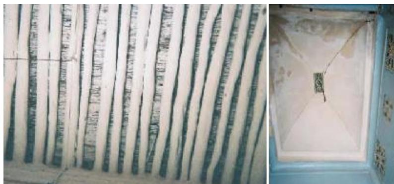
**Fig. 5.** Wood framed floors and edge vaults.
