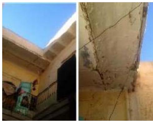
**Fig. 9.** Brick floor supported by IPN metal beams.
