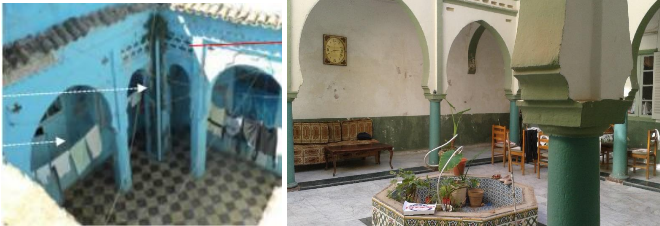
Fig. 4. Typology of porticos in the traditional houses of the medina of Tlemcen.
