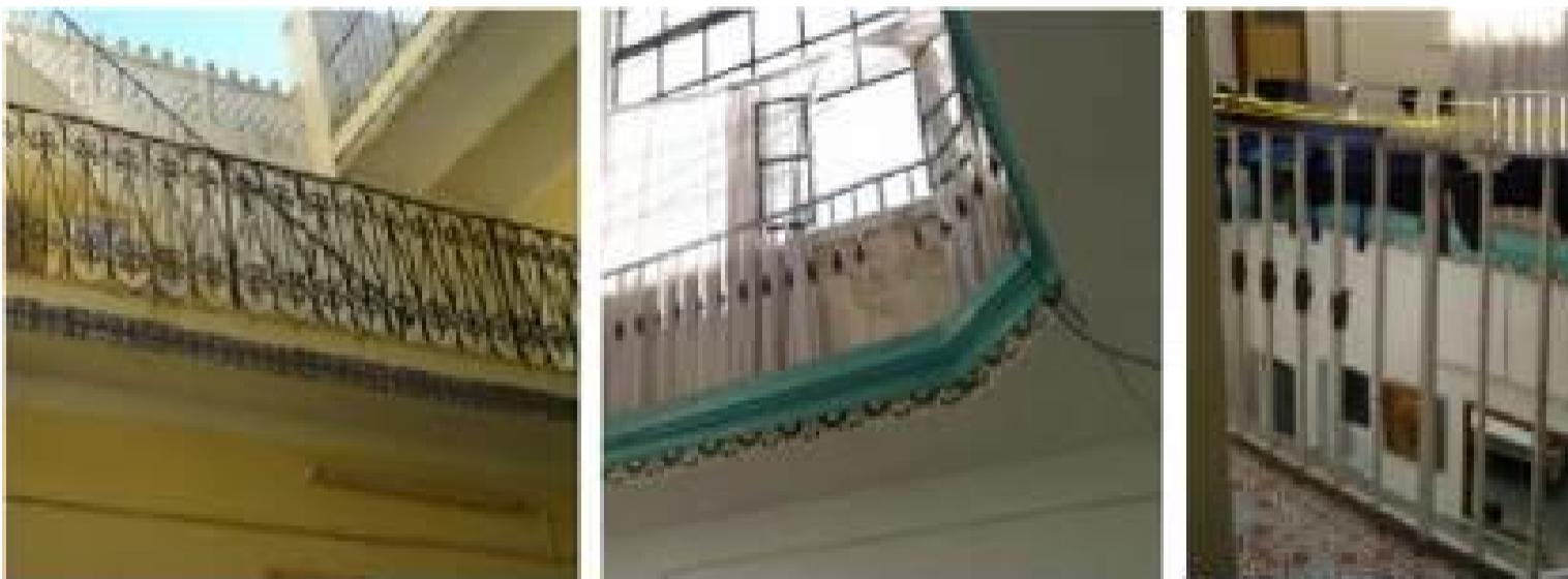
Fig. 13. Wrought iron metal balustrades.
