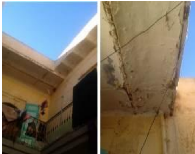
Fig. 9. Brick floor supported by IPN metal beams.
