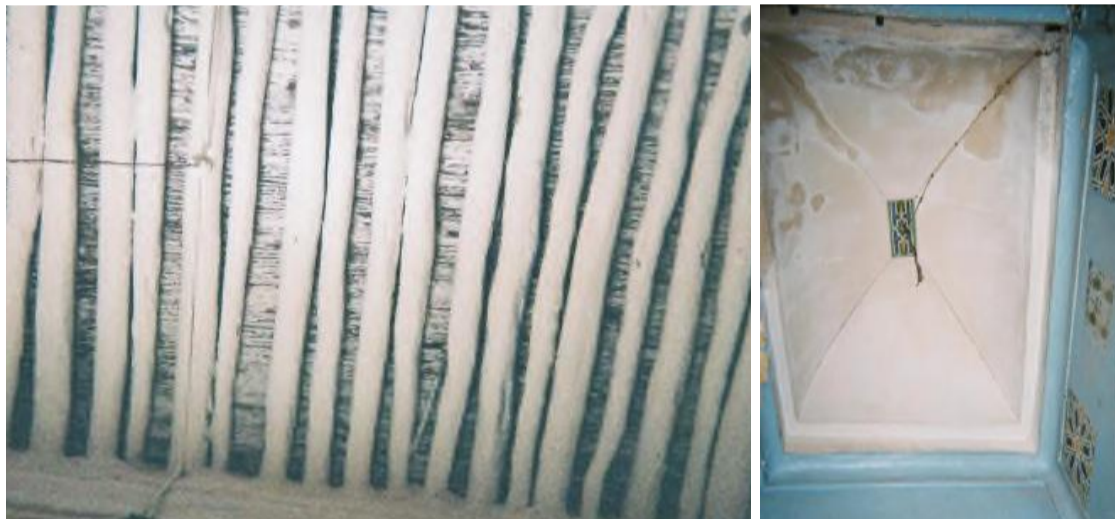
Fig. 5. Wood framed floors and edge vaults.
