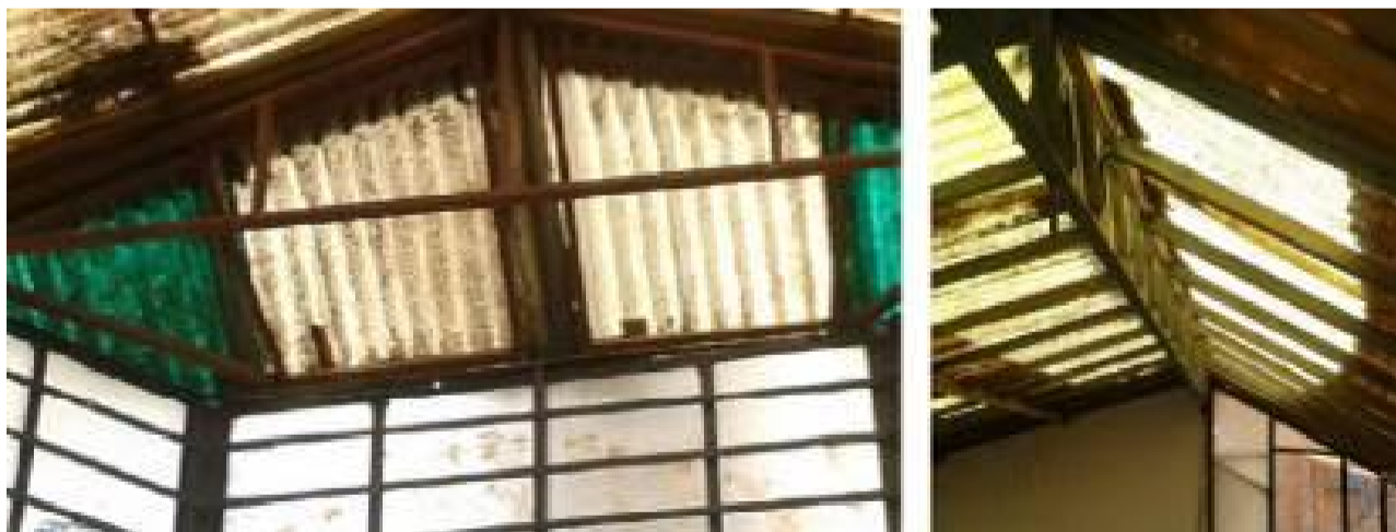
Fig. 10. Patios covered with metal structures.
